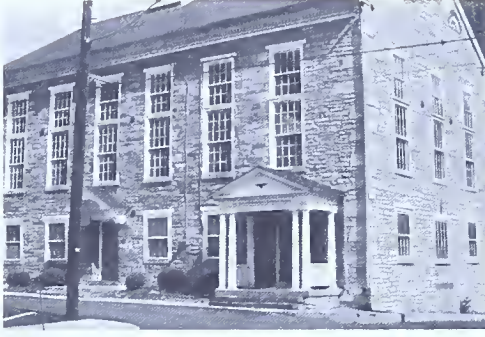
Hummelstown Area Historical Society building (c. 1815) (former Zion Lutheran Church), Rosana Street, Hummelstown; (Ordovician) limestone and dolomite from local quarries in Dauphin County.
